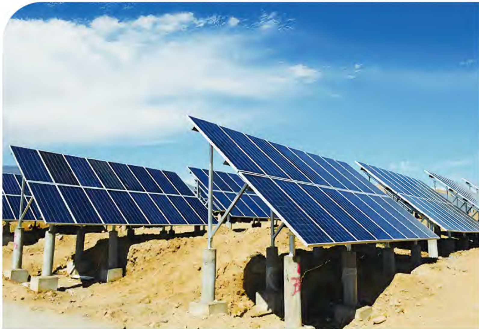
500MW | 甘肃华能海南州 | 固定式支架系统 Fixed Support System in Huaneng Hainan Prefecture, Gansu, 500MW
